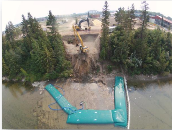
River; Stream Diversion; & Site Isolation
